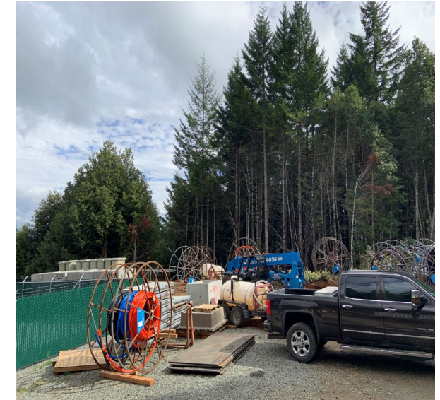
Preparing construction yard
