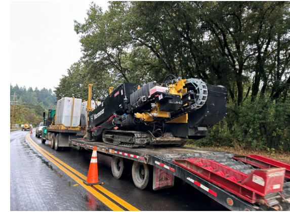
Delivering trenching and vaults
