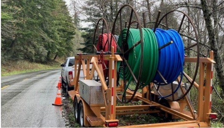
Installing conduit in Humboldt County
