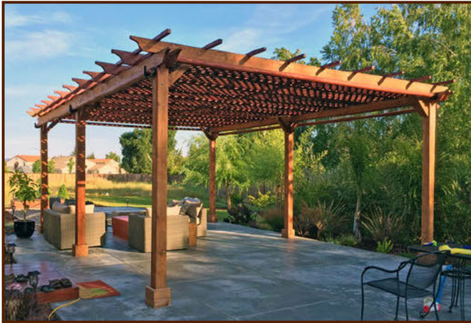
East Side Sierra Shuttle Solar Pergola Progress toward zero carbon!
