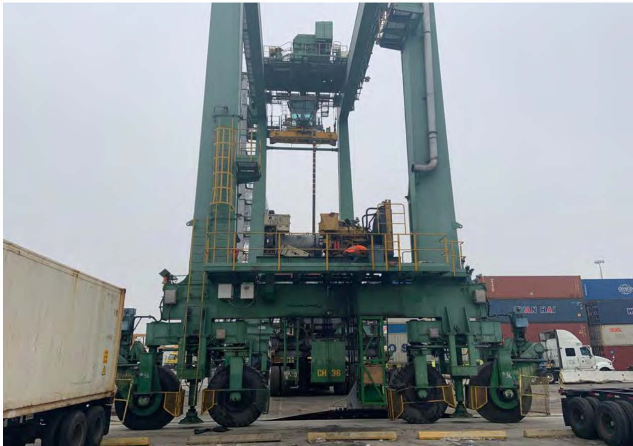
Figure 127. Enclosure removed from RTG crane engine compartment to begin conversion
