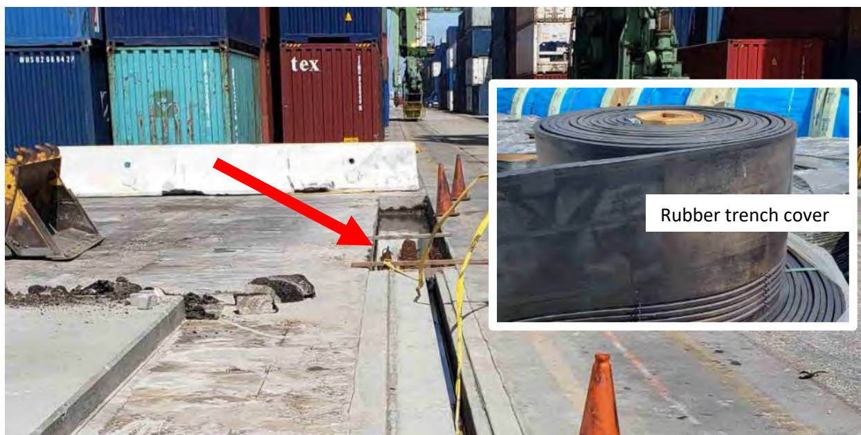
Figure 126. Linear trench being cut and configured for the connection cable
