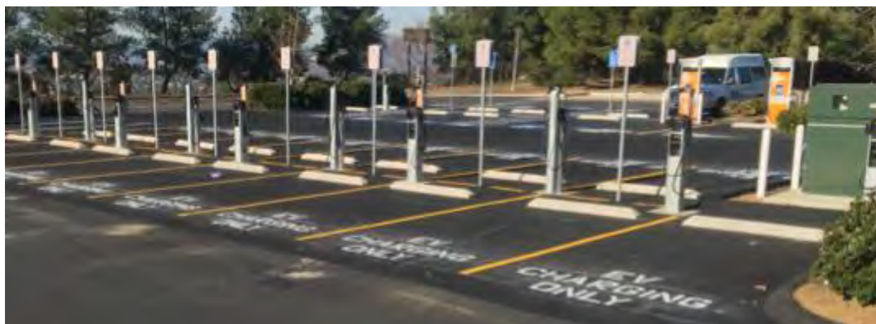
Figure 96. Row of L2 EVSE with DCFCs (ADA L2 EVSE in the background)
