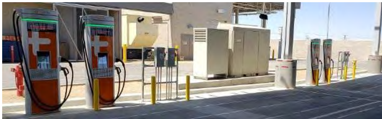
Figure 150. Victor Valley Transit Authority charging station installation
