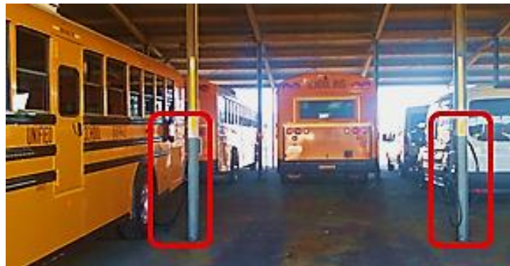
Figure 49. Low-Cost Level 2 Installations, Indoor with Surface-Mounted Conduit
