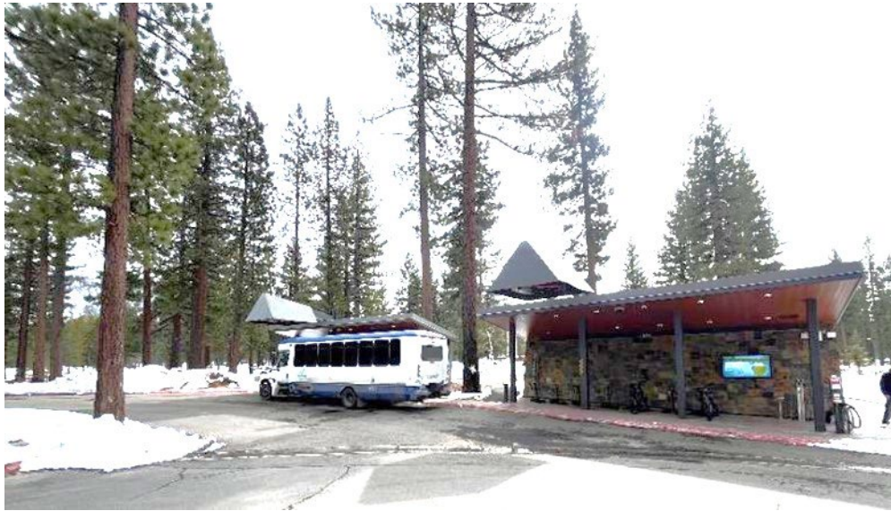
Figure 261. Liberty EV Bus Infrastructure Program LTCC Mobility Hub with Pantograph EV Chargers
