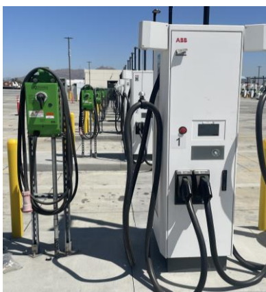
Figure 72. SCE Charge Ready Transport Program Charging Island Supporting TRU and Truck Charging
