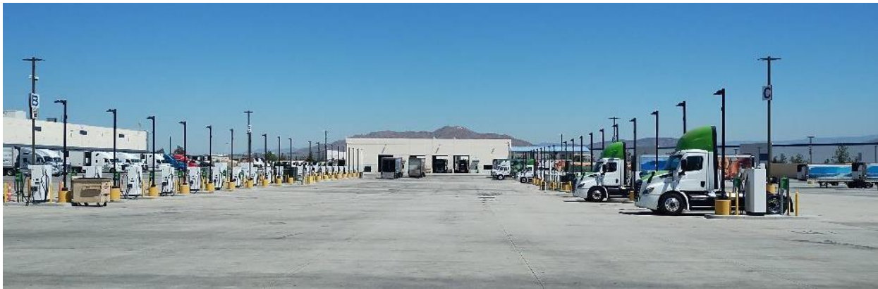
Figure 70. SCE Charge Ready Transport Program Heavy-Duty Truck Yard with 80 DCFC Charging Ports
