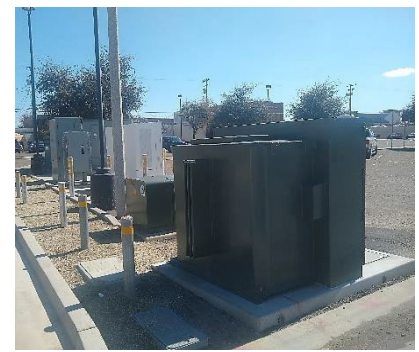
Left to right: Depot fast charger; en route charger dispensers; en route electrical switchgear and transformer
