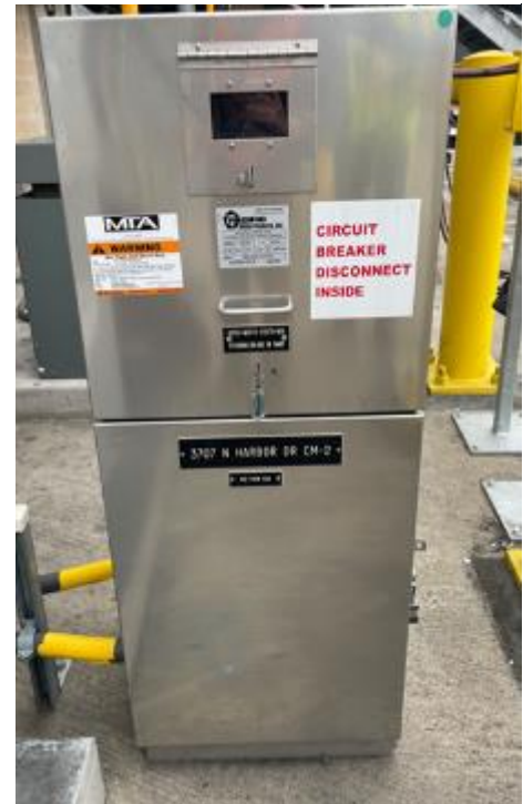
Figure 146. Example of Enclosure Cabinet for Load Research Meters
