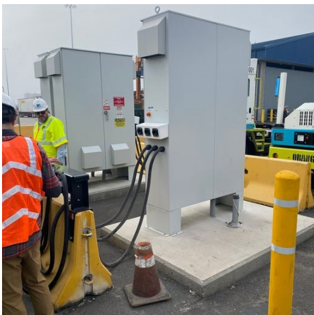
Left: Three-port DCFC dispenser; center: DCFC power cabinet (180 kW); right: electric yard tractor
