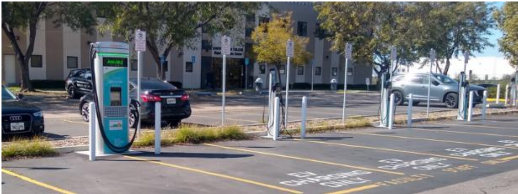
Figure 179. SDG&E Schools and Parks Pilots Examples of DCFC and L2 EVSE with Very High Access to Parking Spaces
