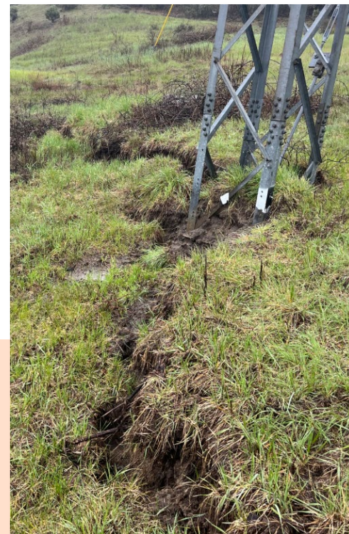
Example of a JIT tower replacement due to imminent landslide hazard.
