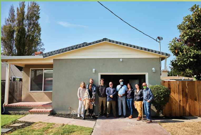
Below: The first home to be completed as part of MCE's Virtual Power Plant in Richmond, CA
