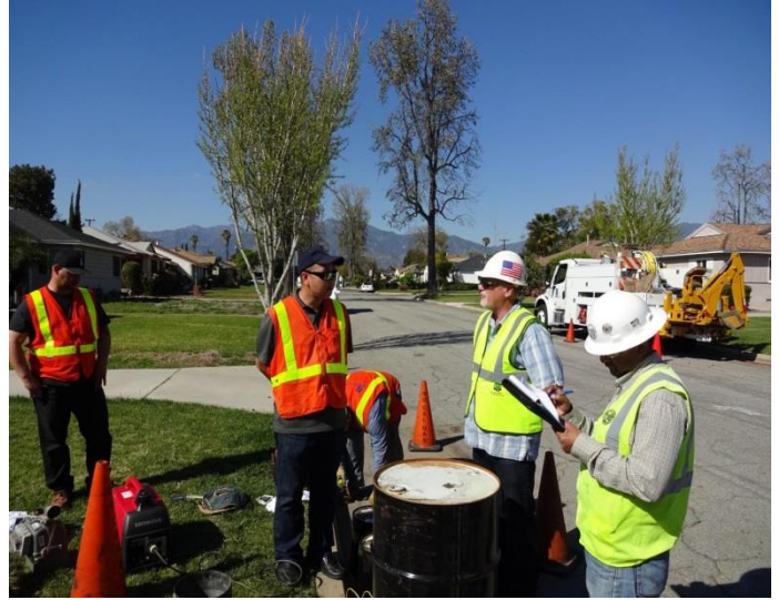
CPUC and utility staff perform gas pipeline safety inspections. CPUC and utility staff inspected hundreds of miles of gas pipeline in 2016.
