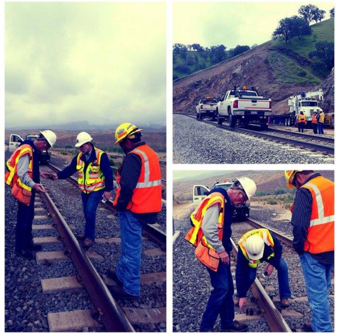
CPUC safety staff inspect railroad tracks in Tehachapi, California. Every year, CPUC staff visually assesses hundreds of miles of rail tracks in California, in addition to inspecting rail crossings and investigating rail safety incidents.
