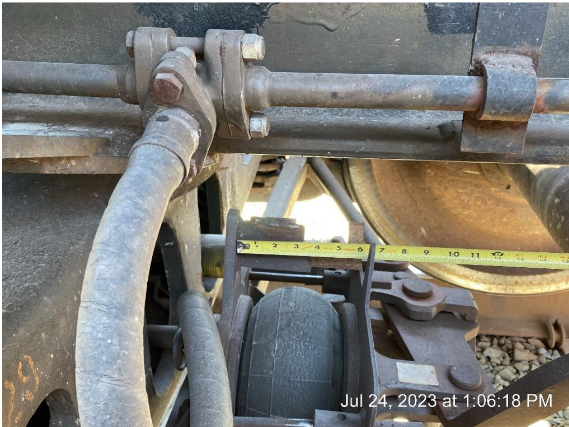
Excessive piston travel found in braking system
