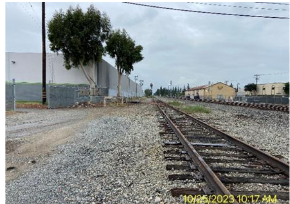
After: Locomotives moved and debris cleared
