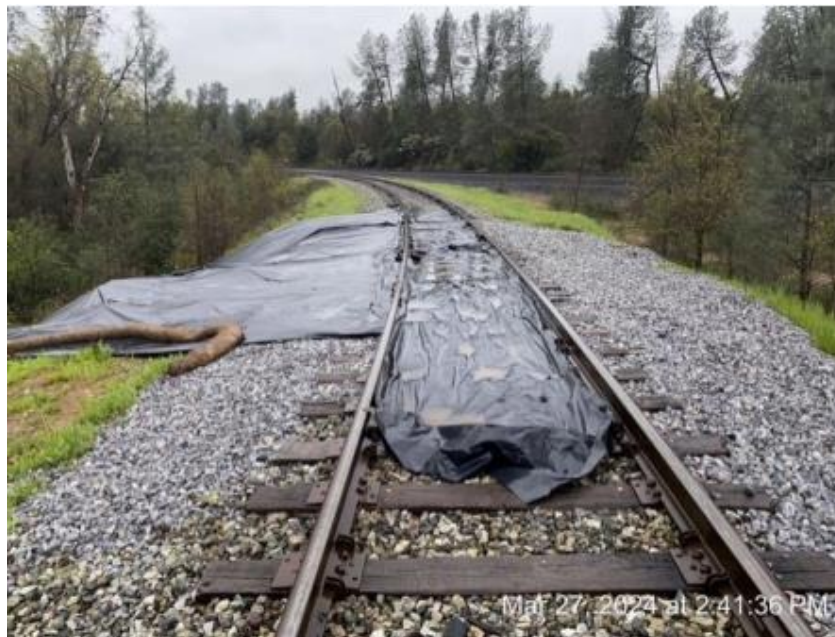
Tarp covering the walkway
