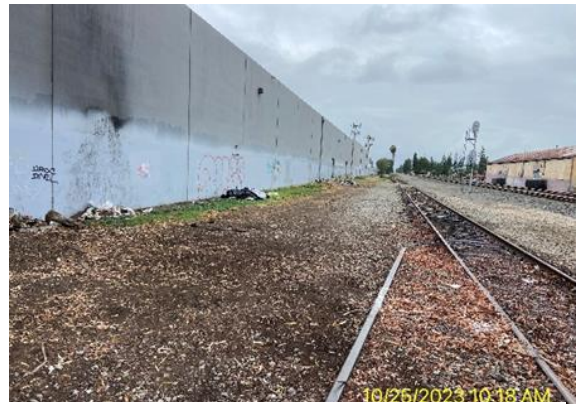
After: Encampment and debris removed from property
