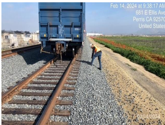
Before: Home Depot track showing incorrect walkway. (118-A) After: Walkway slope corrected.
