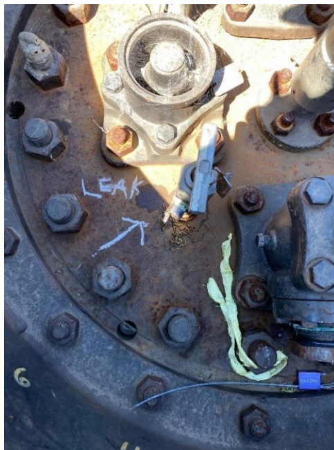
Defective sample line valve creating a leak
