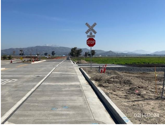
Before: Crossing missing ENS sign, and post not reflectorized.
