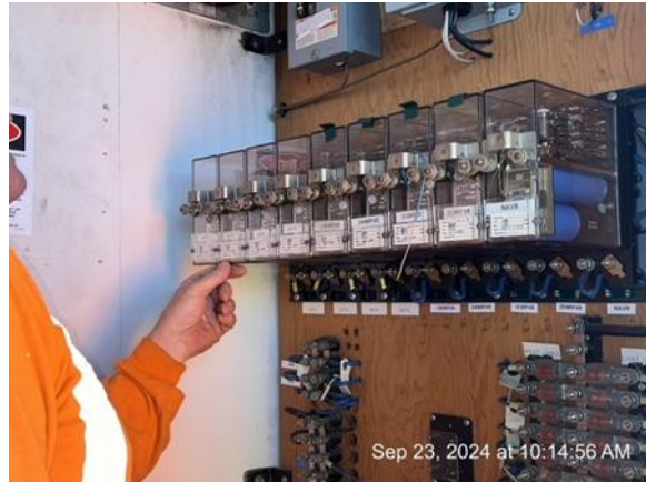
Relays: Verifying the correct relay corresponds with the correct track circuits for the bridge.
