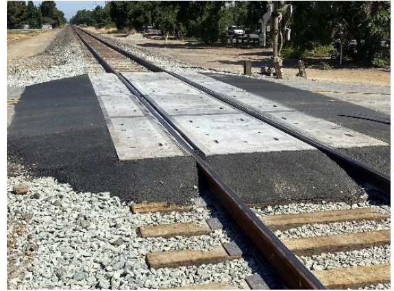
GO 72-B: After: Completely renewed crossing with new track.
