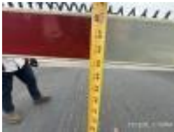
Gate arm corrected to proper height per GO 75-D
