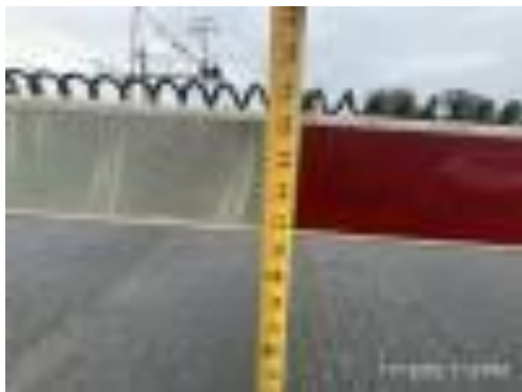
Low gate arm height out of compliance
