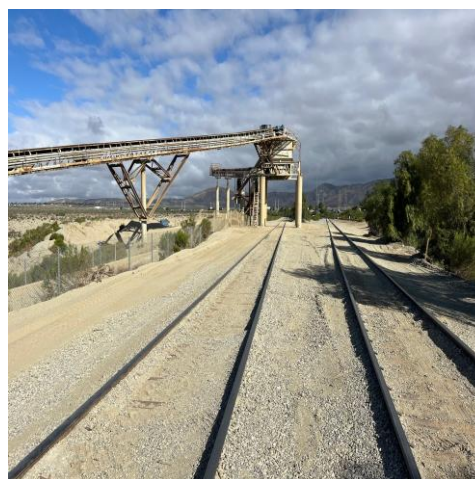
Vegetation removed from walkway
