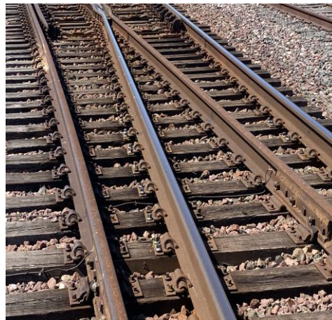
After Fasteners Reinstalled
