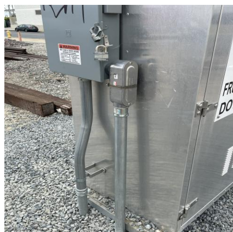
Repaired wire housing.
