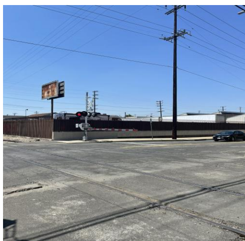
Gates lowered due to false activation.
