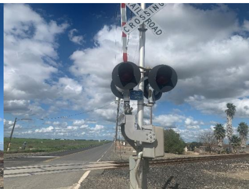
Crossing light repaired
