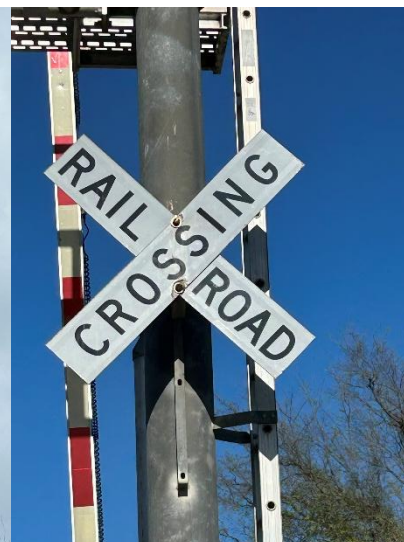
Replaced crossbuck signage
