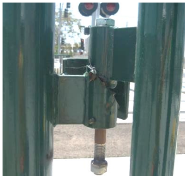
Figure 2.4.5 - Example of Gravity Hinge
