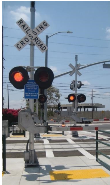
Figure 2.5.2 - Example of a Pedestrian Automatic Gate/Standard 9 Pedestrian Gate
