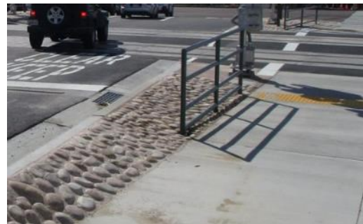
Figure 2.3.14 – Uneven Textured Surface using Rock Blankets (Photo)
