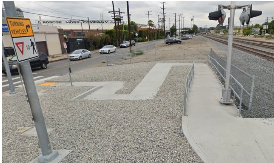
Figure 1.3.1 – Example of Approach Slope and Landing
