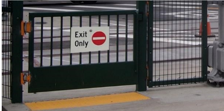
Figure 2.4.6 - Emergency Egress Swing Gate Equipped with a Kickplate
