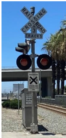
Figure 2.5.1 - Flashing Light Signal Assembly/Standard 8 Warning Device
