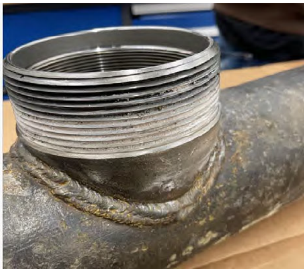
Figure 3. Post Incident Photo- 4” Mueller Line Stopper without installed cap and completion plug (side view)
