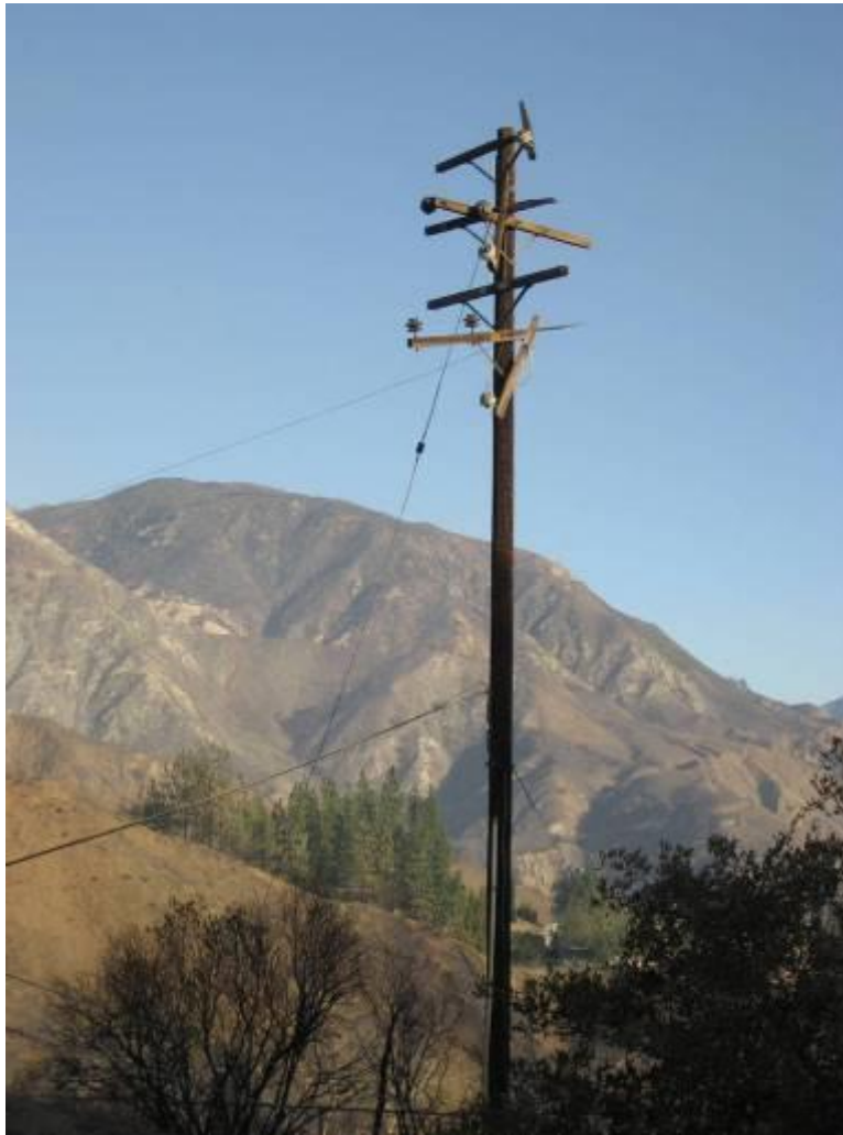
Photo 2 Damaged Cross-arm
