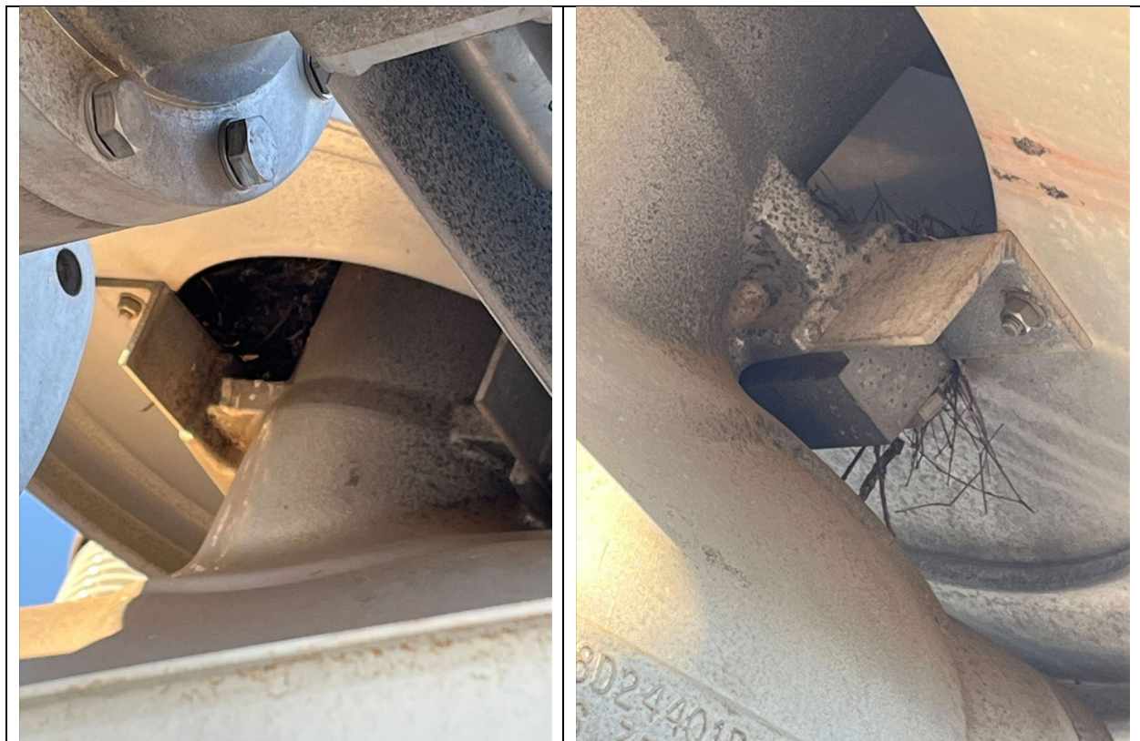
3.2. Bird nest in CB102 current transformer.
