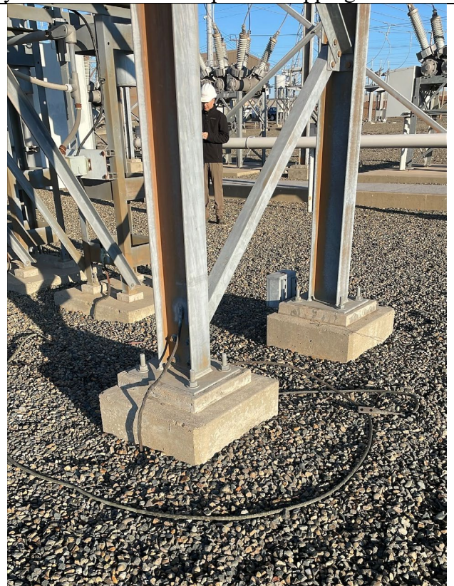
3.4. Exposed ground cable in the 69 kV yard near switch 7222 poses a tripping hazard.
