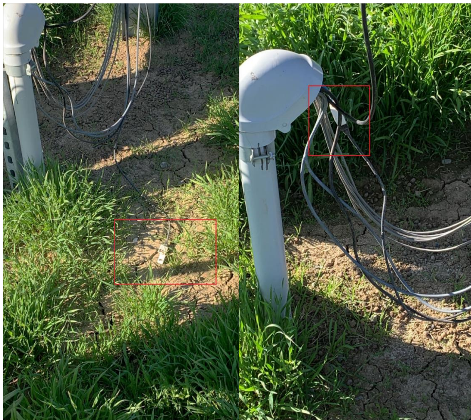
Figure 6 Heliostat Unconnected Ethernet (Left) Corrected (Right)
