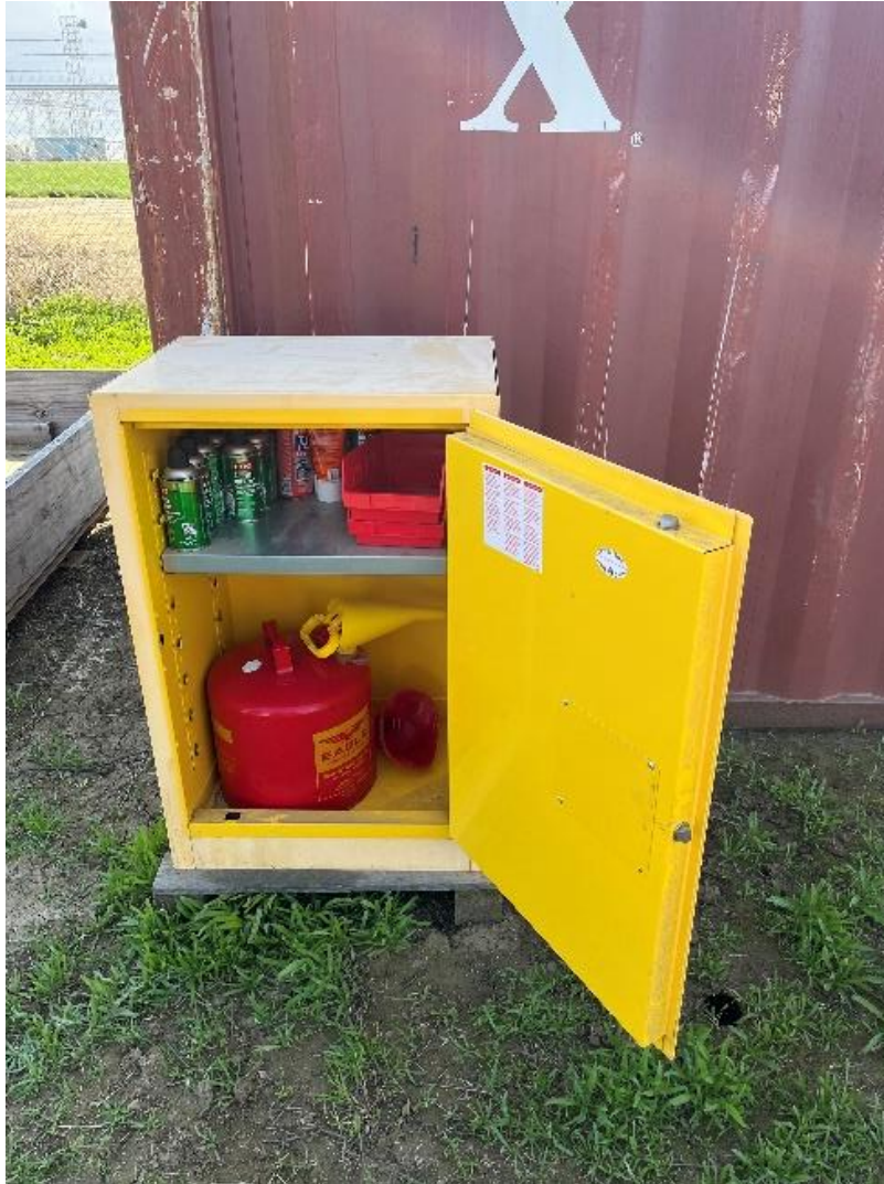
Figure 2 Flammable Storage Door Ajar
