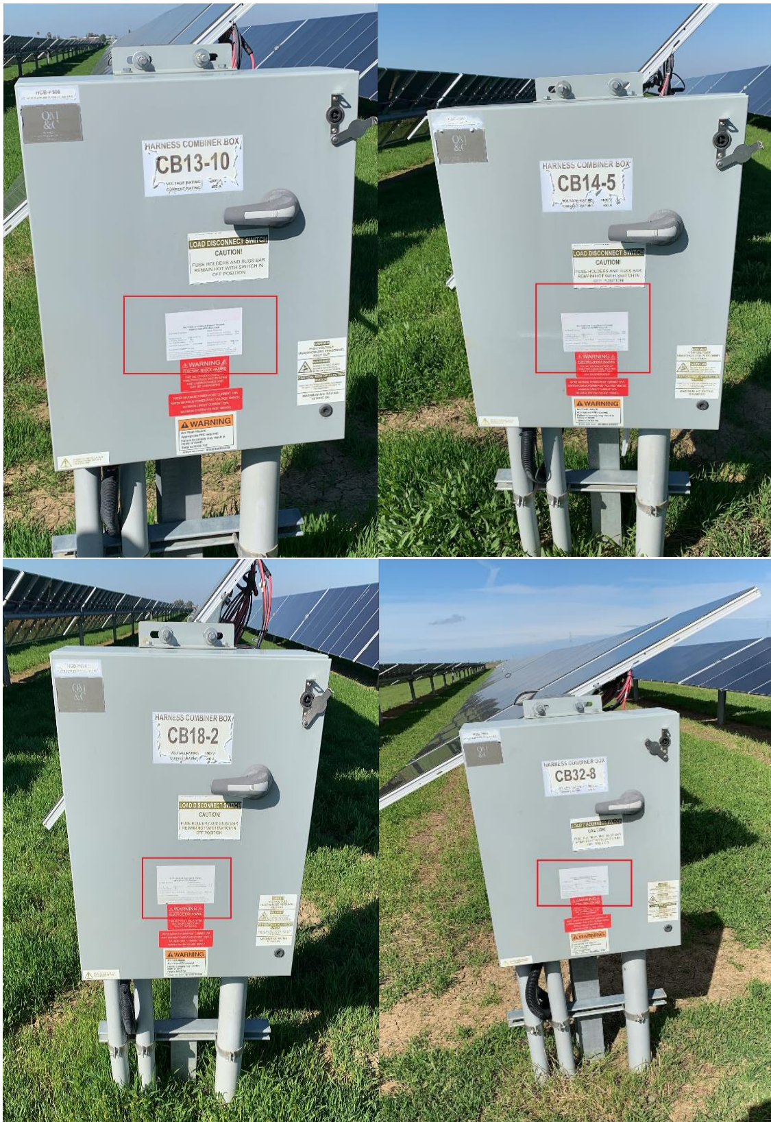
Figure 4 Combiner Box Deteriorated Danger Labels
