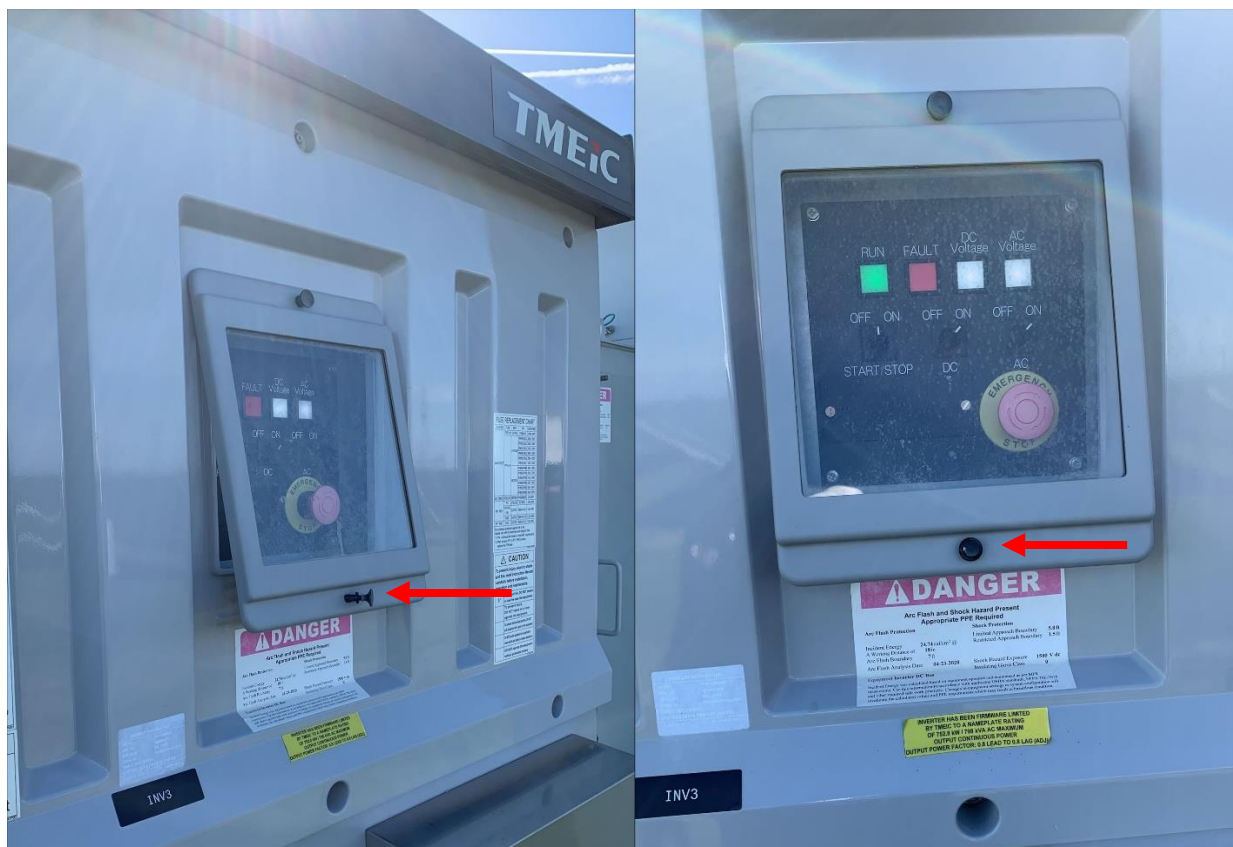
Figure 8 Inverter 21(Left) and Inverter 34(Right) Cover Ajar with broken Pin
