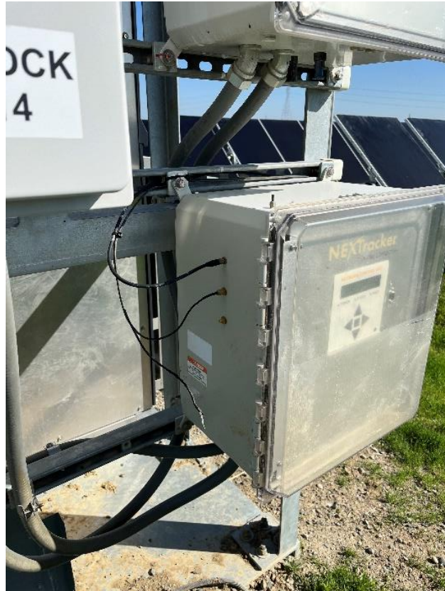
Figure 5 Broken connection on inverter communication device
