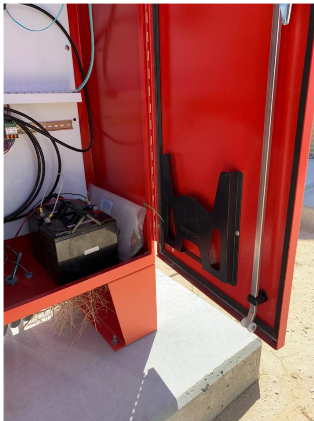
Figure 8: Fire alarm control cabinet with no ERP.
