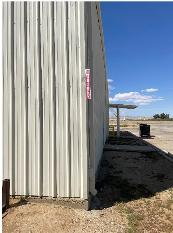
Figure 4: Fire extinguisher sign on outside of the storage warehouse with no fire extinguisher.
