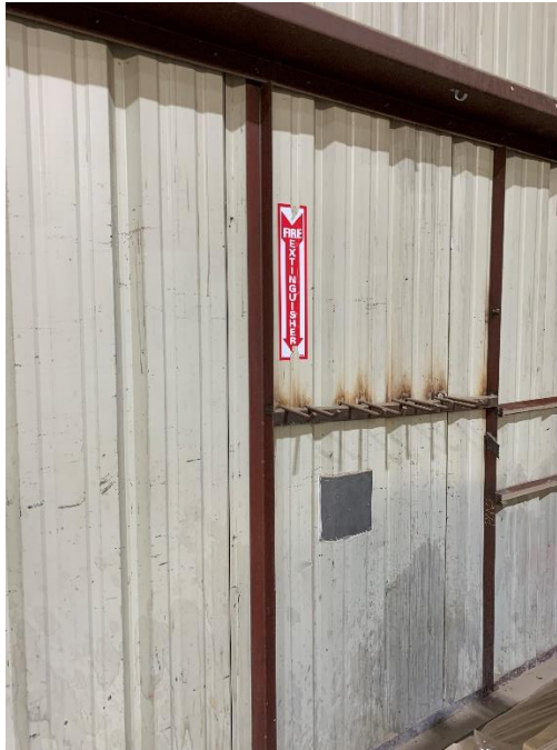
Figure 5: Fire extinguisher sign inside of the storage warehouse with no fire extinguisher.
