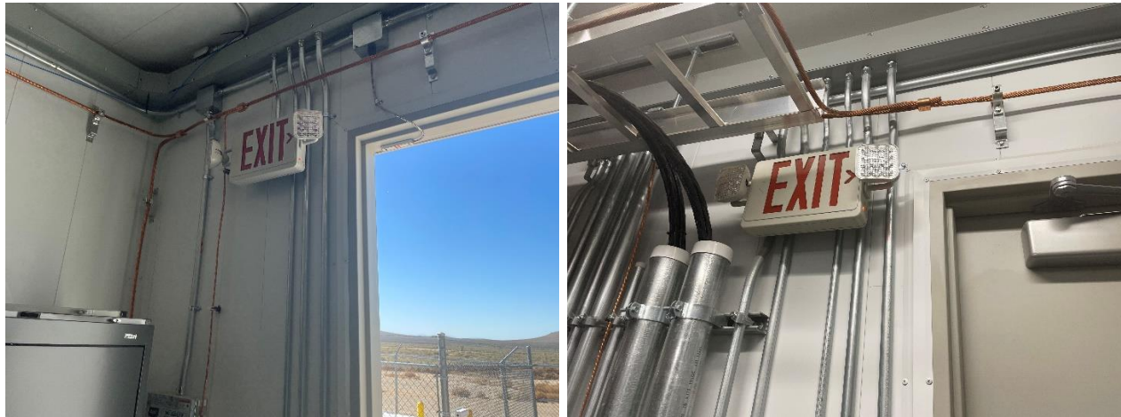
Figure 3: Nonfunctioning emergency lighting in substation.
