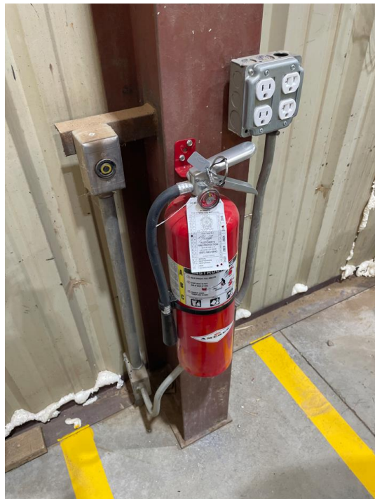
Figure 7: Fire extinguisher with a missing monthly inspection tag.
