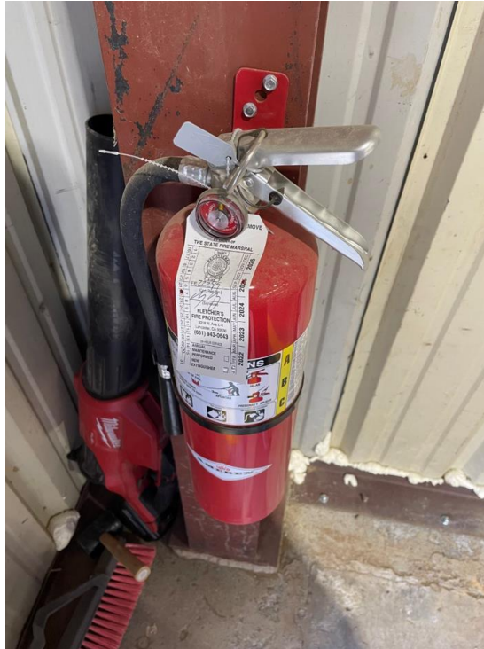
Figure 6: Fire extinguisher with a missing monthly inspection tag.
