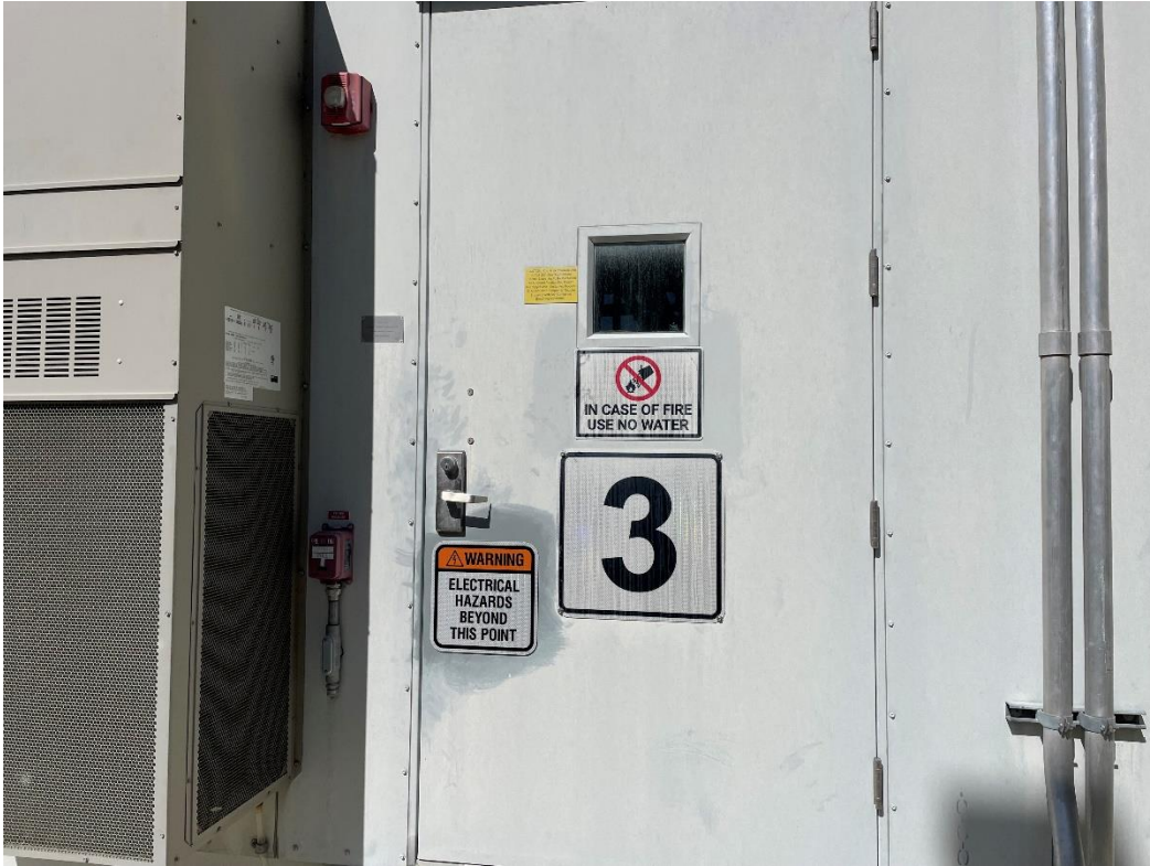
Figure 3: Electrical Package entrance without, and with, electrical hazard identification signage
