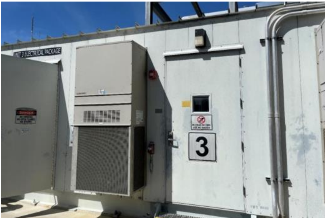
Figure 2: Electrical Package door without, and with, electrical hazard identification signage
