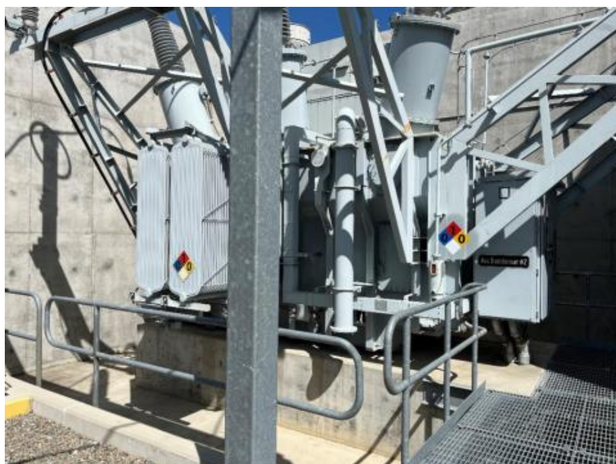
Figure 5: Corrected NFPA Placards
