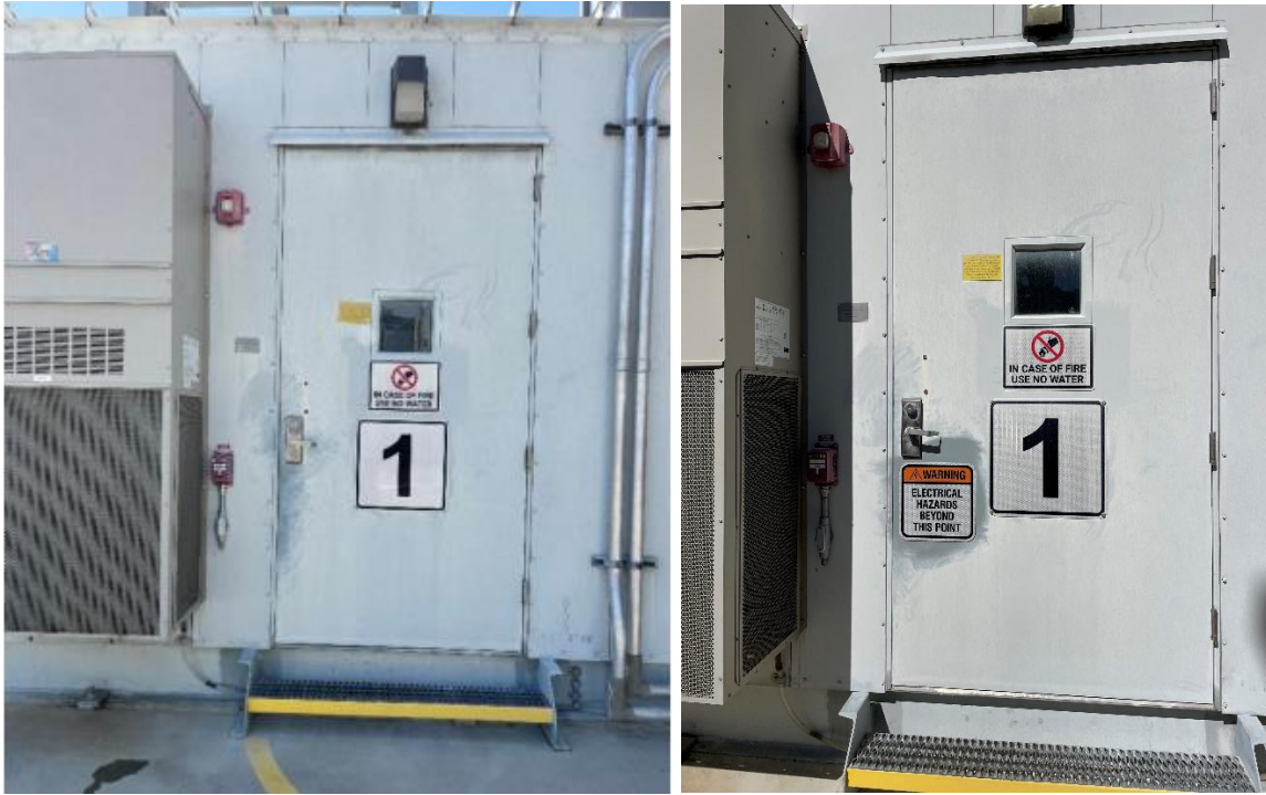
Figure 2: Electrical Package door without, and with, electrical hazard identification signage
