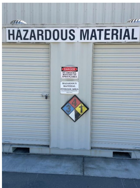
Figure 6: Hazardous Material Storage NFPA sign was updated to reflect the highest level stored inside the container at time of ESRB visit.
