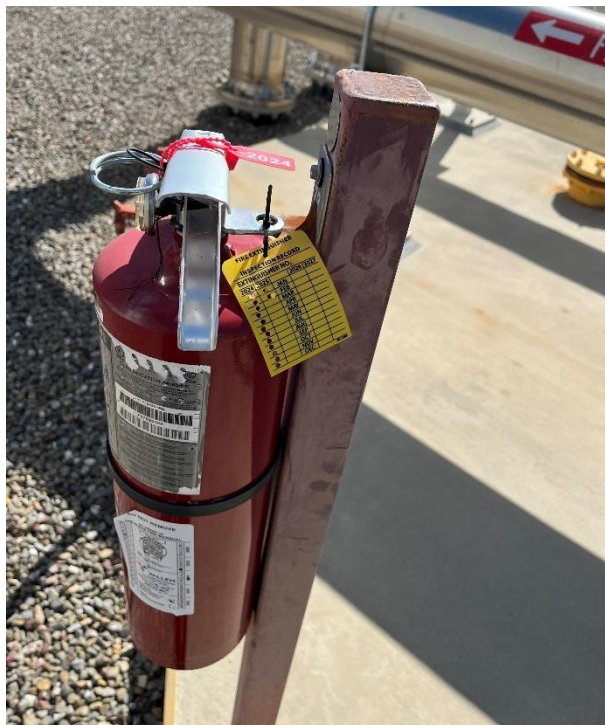
Figure 9: Fire Extinguisher 26 (Water Tank) missing March Inspection
