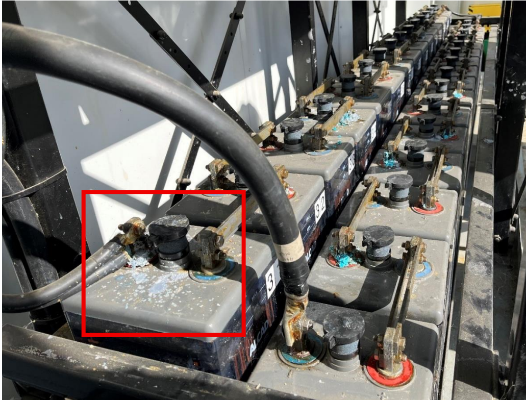
Figure 11: Corrosion on Lead-Acid Battery Terminals
