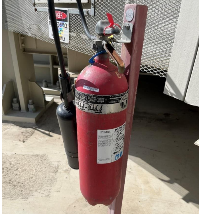
Figure 8: Fire Extinguisher 090 (Unit 4 Stack) with no State Fire Marshal Sticker
