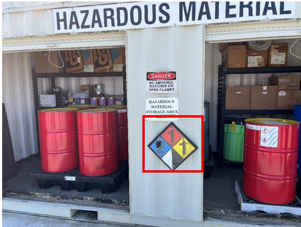
Figure 7: Hazardous Material Storage area does not have the maximum rating of stored contents
