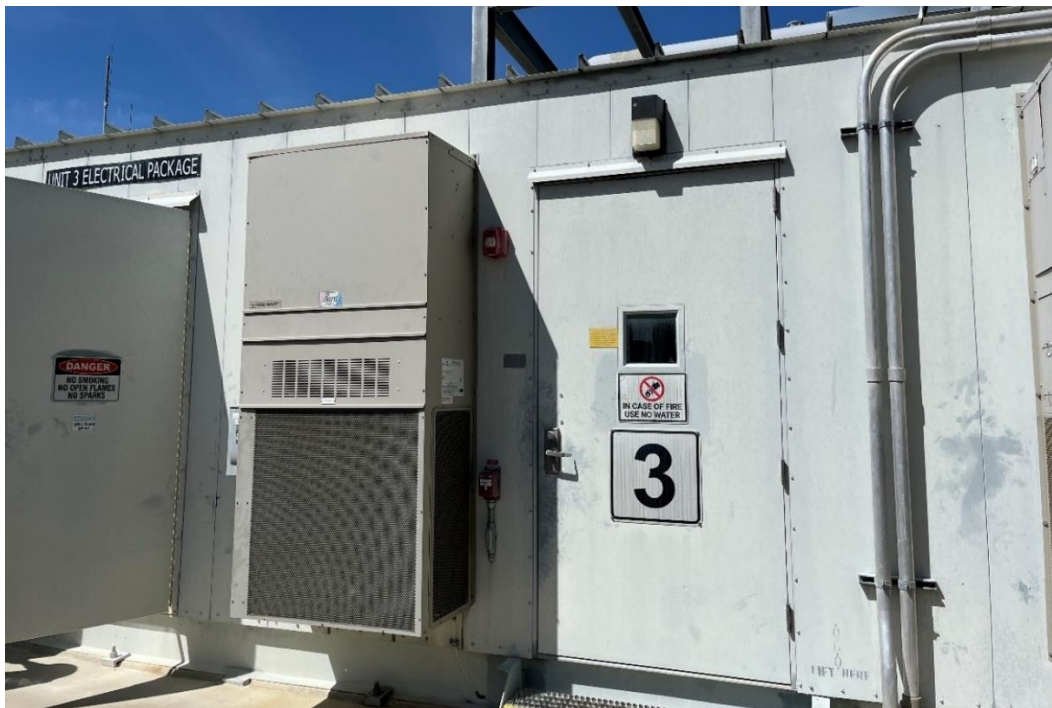
Figure 3: Electrical Package entrance without electrical hazard identification signage
