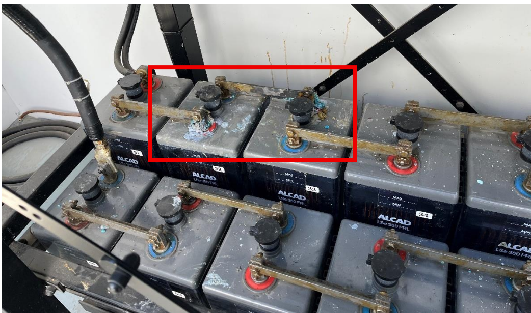
Figure 12: Corrosion on Lead-Acid Battery Terminals
