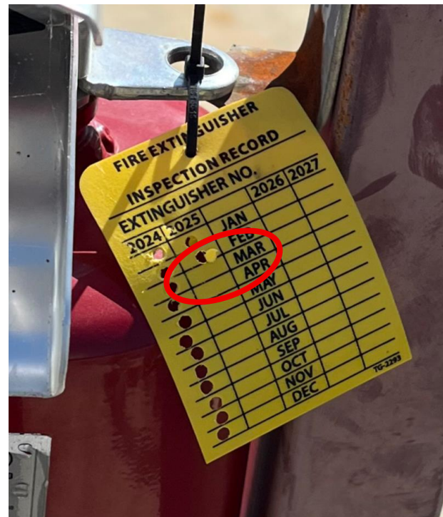
Figure 9: Fire Extinguisher 26 (Water Tank) missing March Inspection
