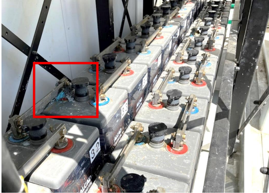
Figure 13: Corrosion on Lead-Acid Battery Terminals
