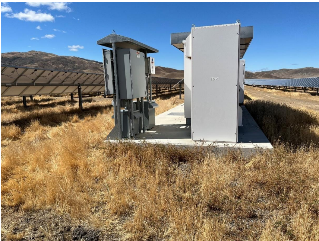
Figure 3: Vegetation growth around Inverter Skid
