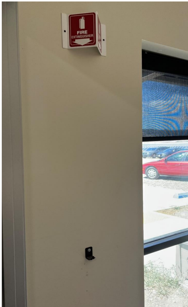
Figure 16: Fire extinguisher missing
