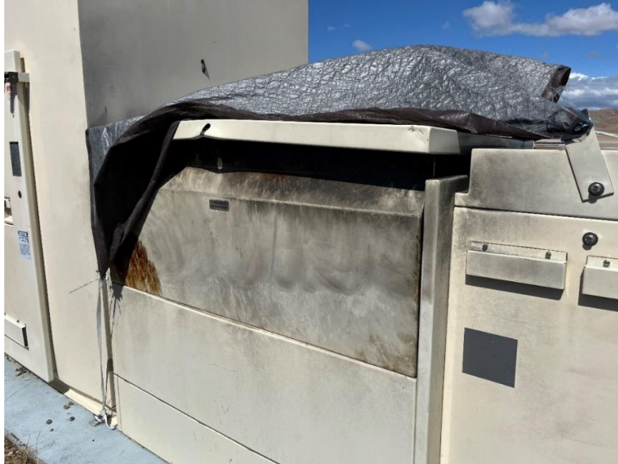
Figure 4: Switchgear 2 – April 2025 Fire Point of Origin
