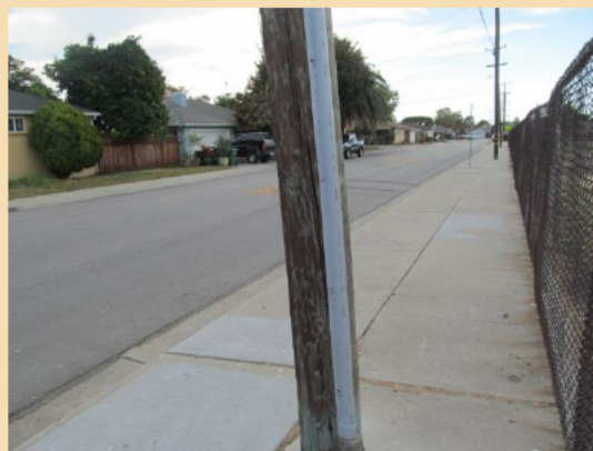
After: 1.5 inch u-shaped molding installed over existing wood molding
