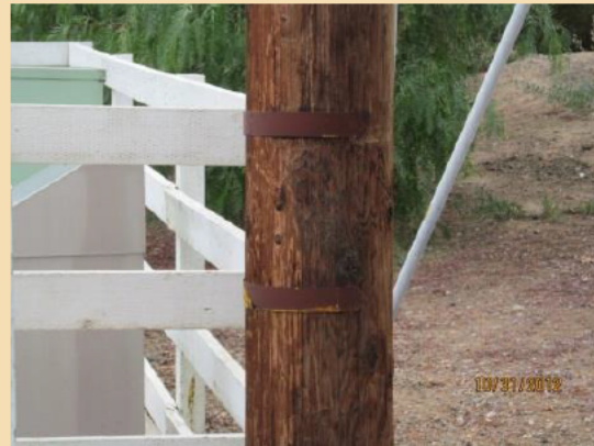
At this Location: Visibility strips painted brown (3 rd visibility strip located above not shown in picture)
