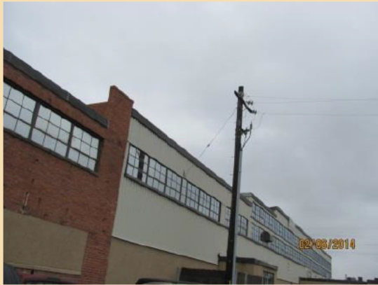
At this Location: Acceptable down guy attached to building, no marker required.
