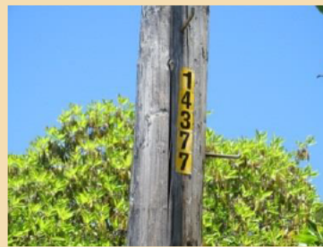
After: Minor work completed, operating number applied below operating position.
