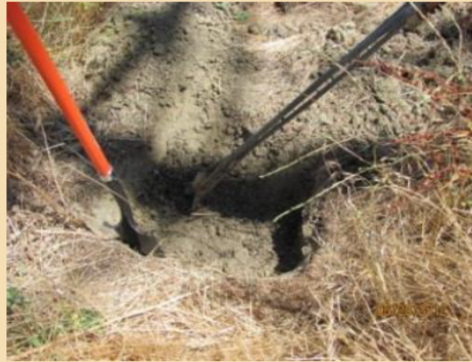
After: Vegetation cleared from anchor
