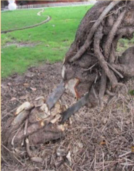
Anchor buried by roots
