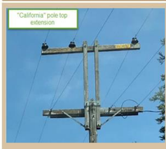
Example: "California" pole top extension
