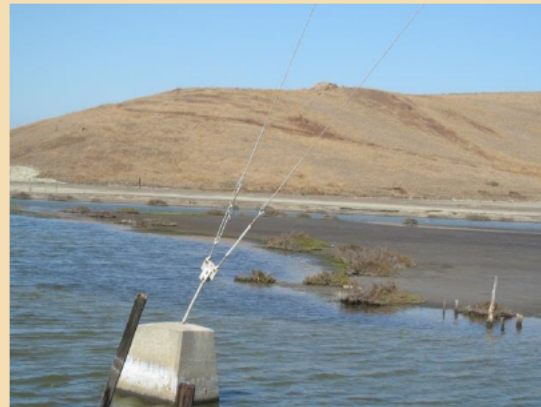
At this Location: Acceptable down guy in marsh, no marker required.
