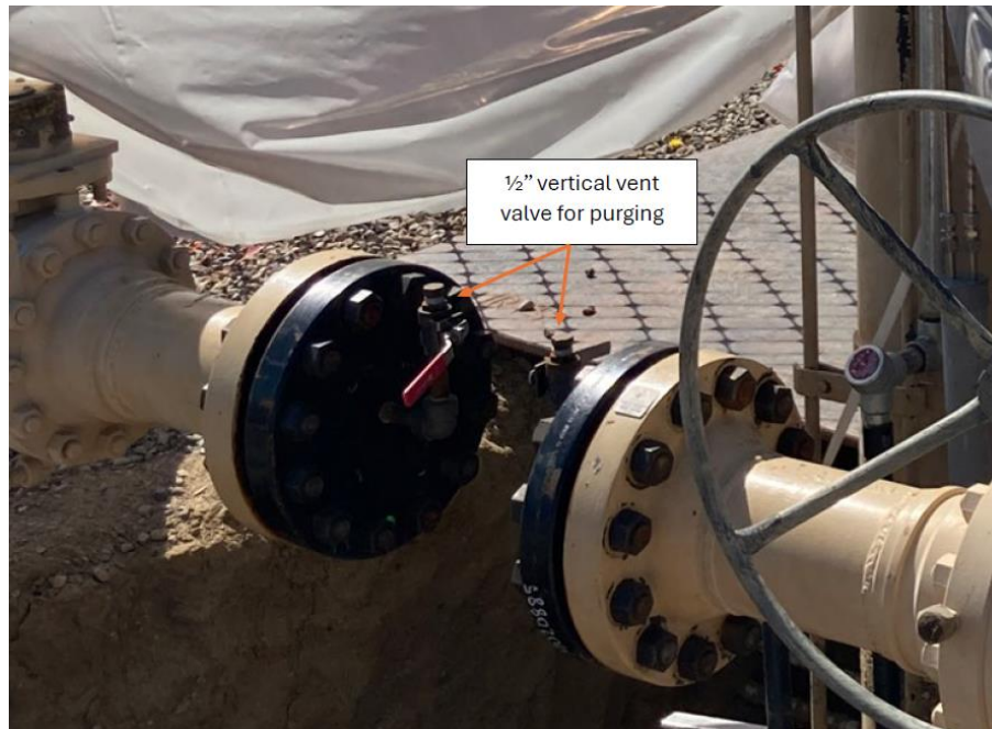
Figure 1: Half-Inch Diameter Vertical Vent Valve Intended for Purging At V-78
