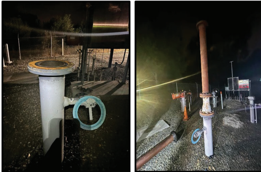
Figure 37: Blowdown Riser locations before stack added (after, on right)
