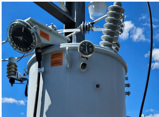
6.3. Voltage Regulator 3 has negative nitrogen pressure.
