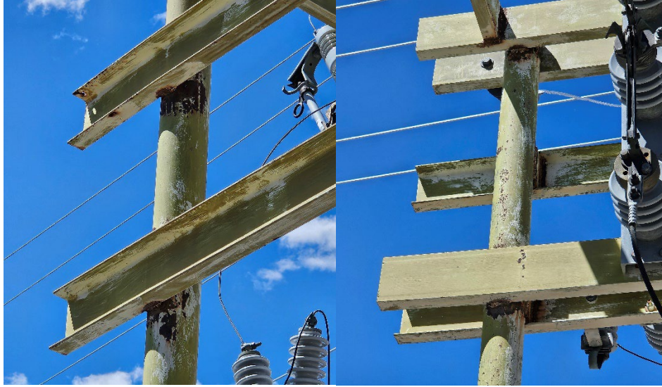
7.2. Recloser H303 has an oil leak.
