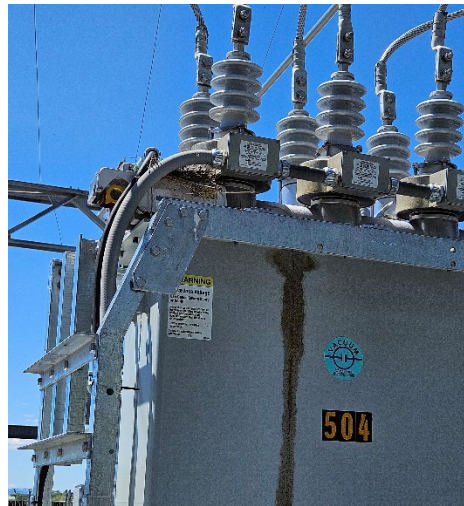
6.3. Voltage Regulator 3 has negative nitrogen pressure.
