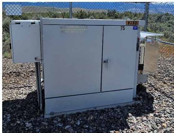
7.3. The Modulation Transformer is missing a high voltage sign.
