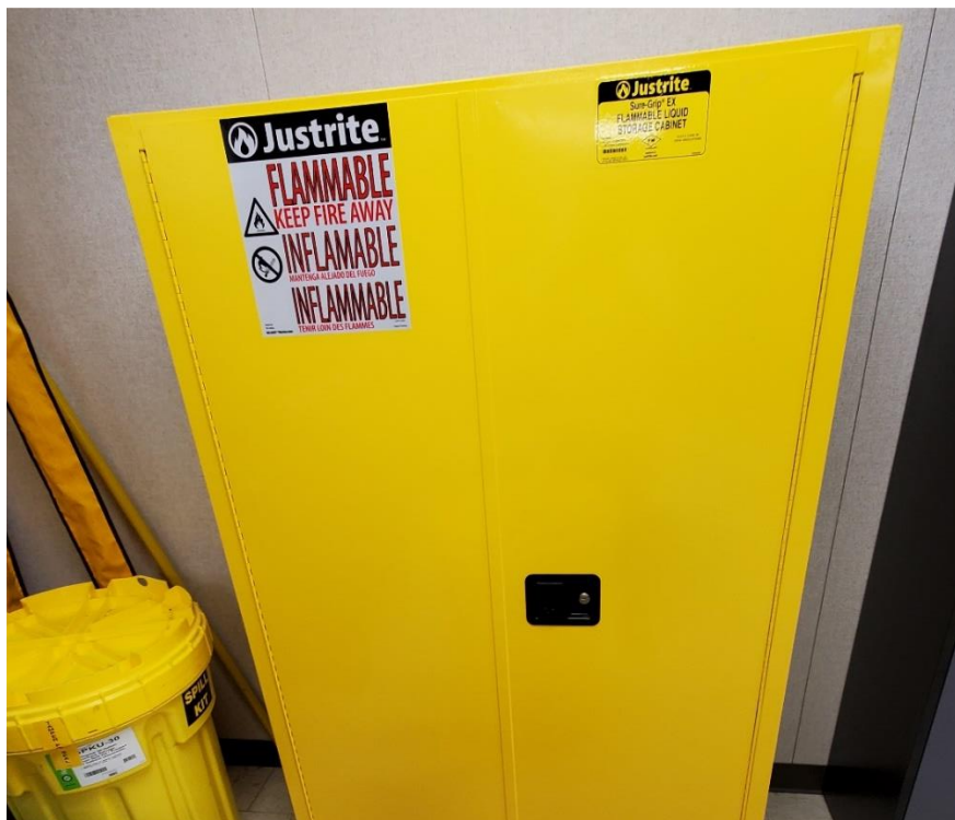
Figure 3: Missing NFPA sign (fire diamond) on Flammable Material Cabinet.
