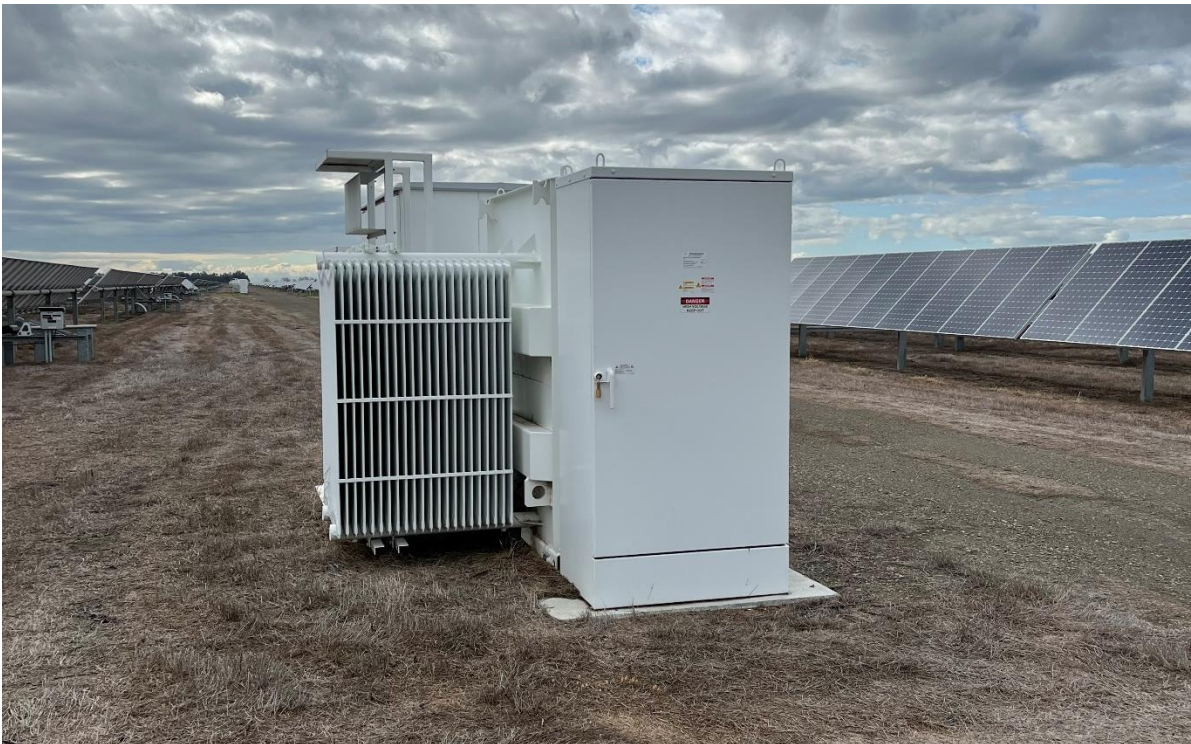
Figure 7: Invasive Loose Vegetation
