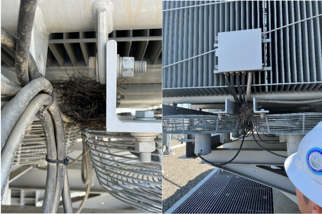
Figure 10: Bird Nest under Transformer Radiator Fins
