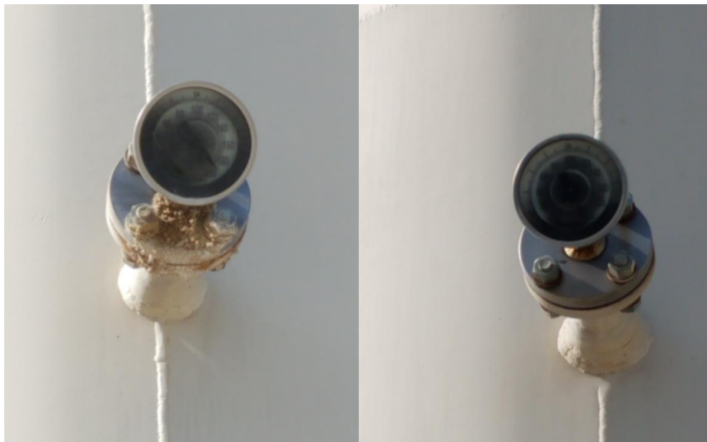
Figure 24: HRC-CIRC water gauges have film making them illegible.
