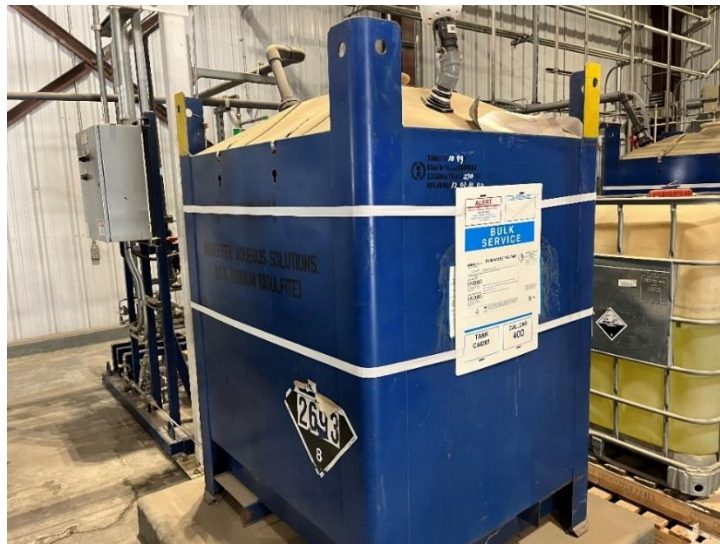
Figure 3: Permacare PC 7408 Stored at Sunrise Power
