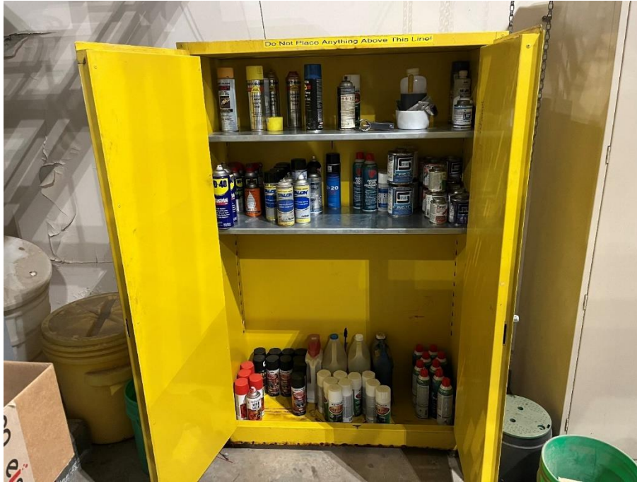
Figure 14: Flammable storage without self-closing doors.
