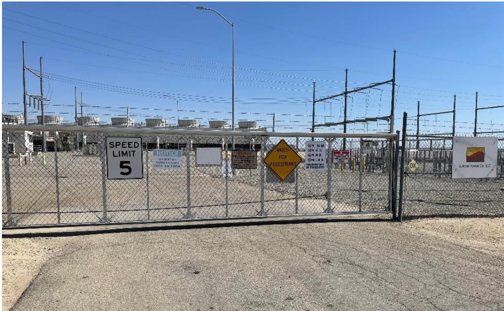
Figure 32: The main gate does not have an NFPA hazard diamond to indicate hazards present at the Plant.
