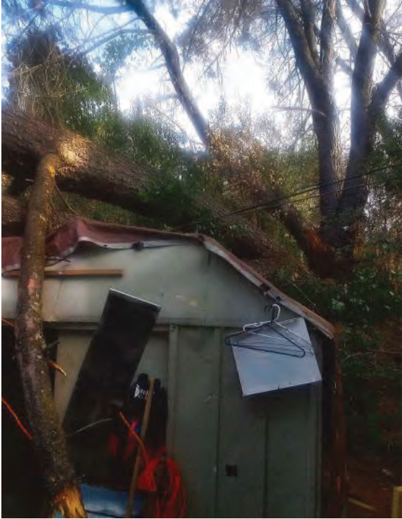
Figure 1: In Oroville, Butte County, a fallen tree hit a shed and cable wire. The tree also came into contact with the service drop (not shown).
