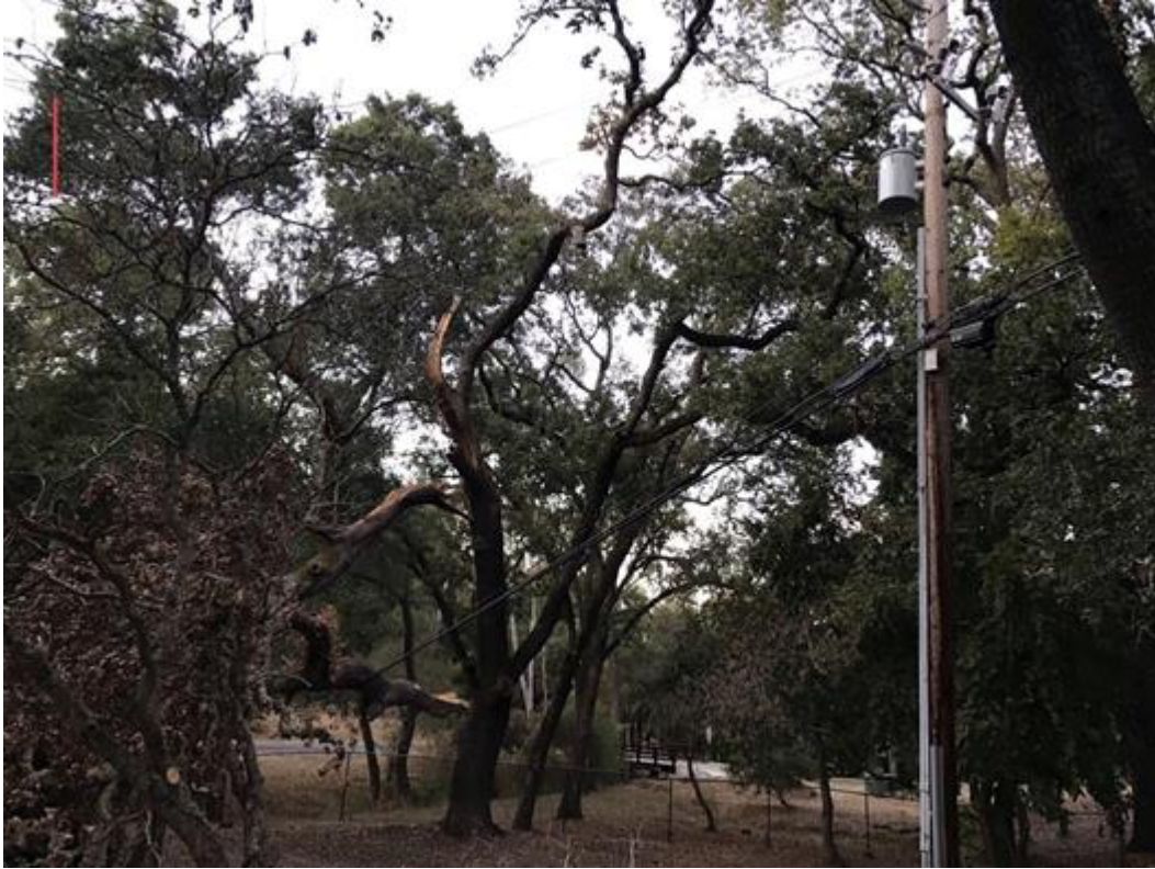
Figure 8 – In Saratoga, Santa Clara Branch Fell Onto Communication Lines
