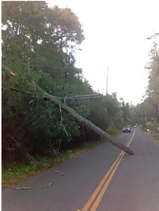
Figure 7: In an unincorporated area of Sonoma County. Tree failed and brought down conductor
