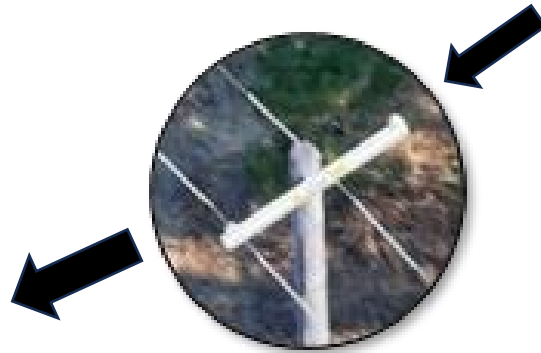
Damage to Equipment
