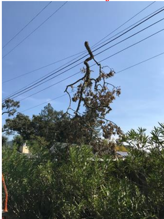
Figure 4 – In Calistoga, Napa County Branch Flew Into Primary Conductors
