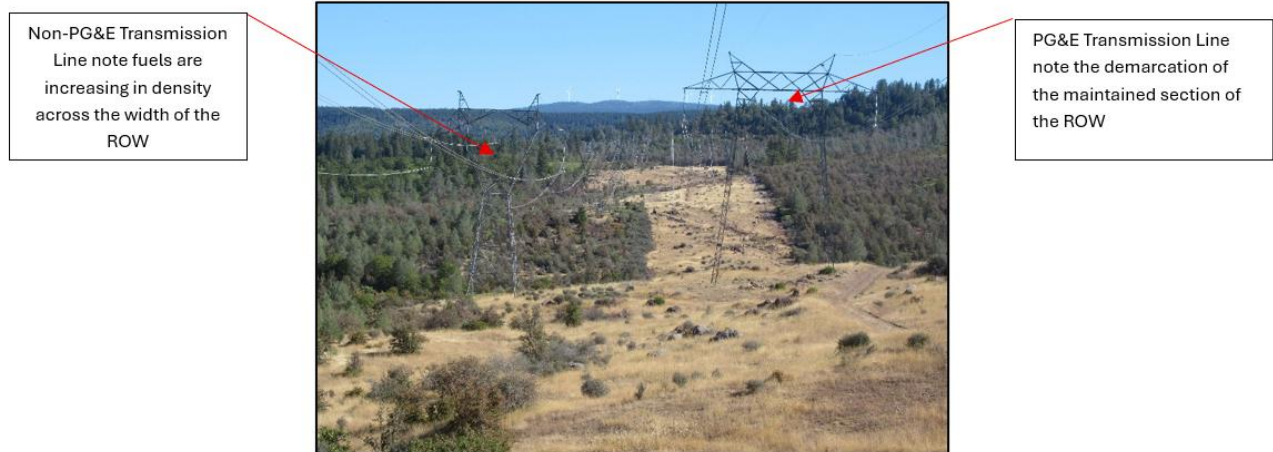
Figure 26: Non-PG&E Transmission Line (left) PG&E Transmission Line (right) note fuel density on left
