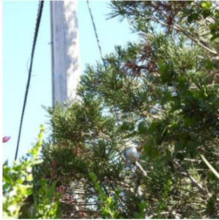
Strain / abrasion on service conductor
