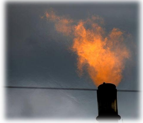
Landfill gas, consisting primarily of methane, is produced via biological breakdown of waste material. Methane is required to be combusted (flared) before being released to the atmosphere for safety and environmental reasons. Methane has a high GHG potential and is highly flammable.
