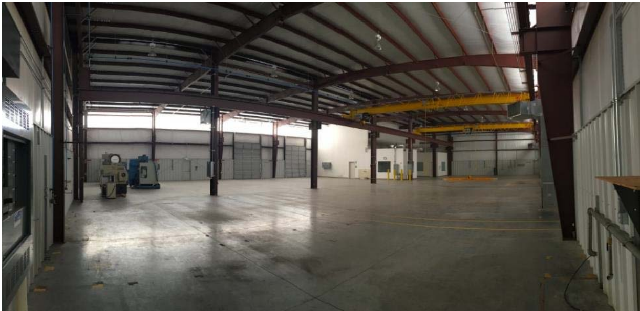
Figure 6— Warehouse Indoor View
