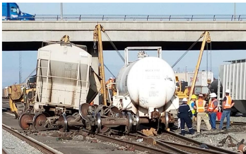
Cleanup activities near Riverside Avenue overpass
