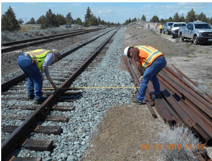
CPUC inspectors taking a measurement
