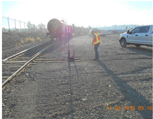
Same area after resurfacing with properly sized ballast
