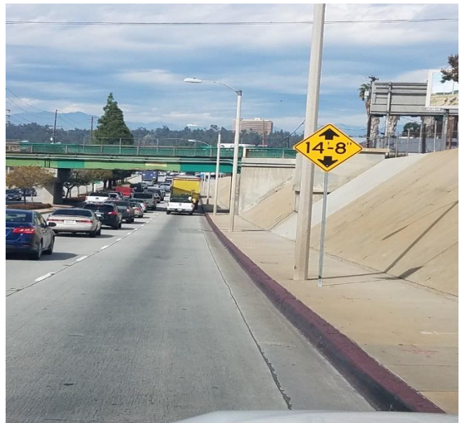
New clearance sign, east side of Azusa Avenue, looking north
