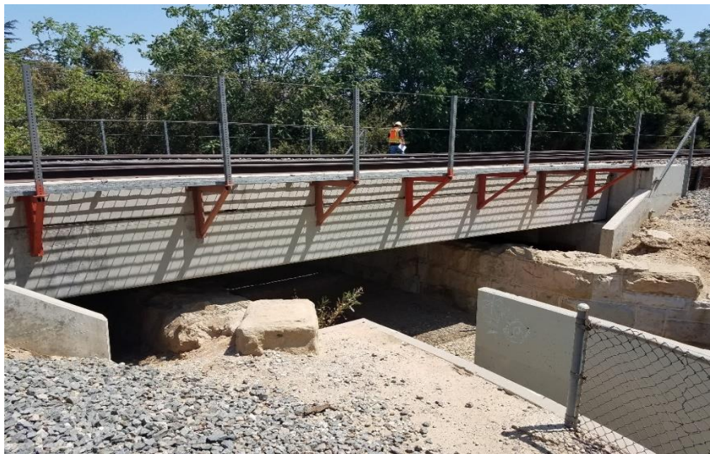
CPUC inspector inspecting a railroad bridge
