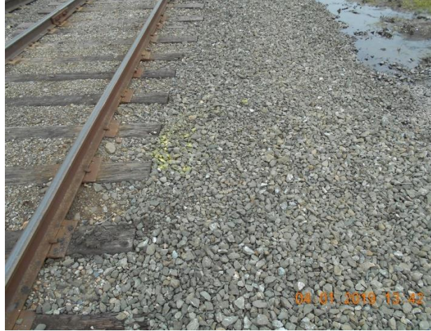
Walkway after hole filled in and surface compacted
