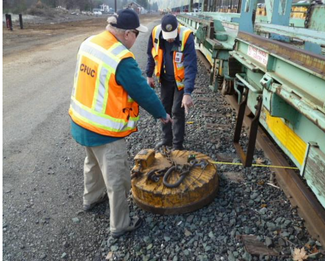
CPUC inspectors identify a large magnet in the walkway during a focused inspection
