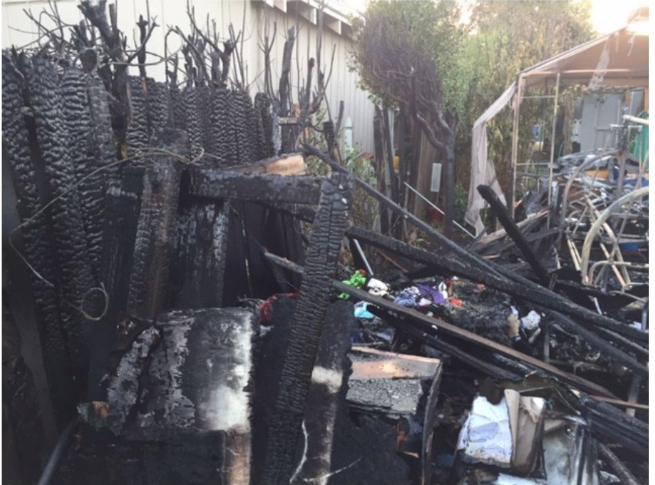
Figure 4: Fire 4 at 258 Barker Street
