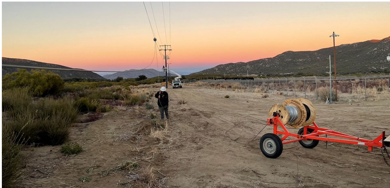
Figure 1: Deployment of Anza Electric's CASF Connect Anza project, Riverside County
