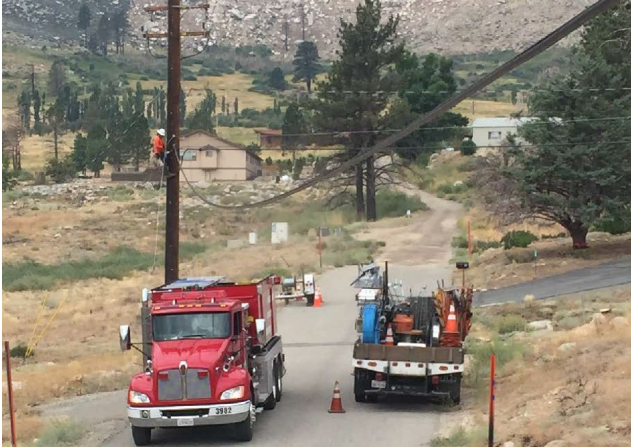
Figure 2: Deployment of Race Telecommunications’ CASF fiber-to-the-premises project in Mono County
