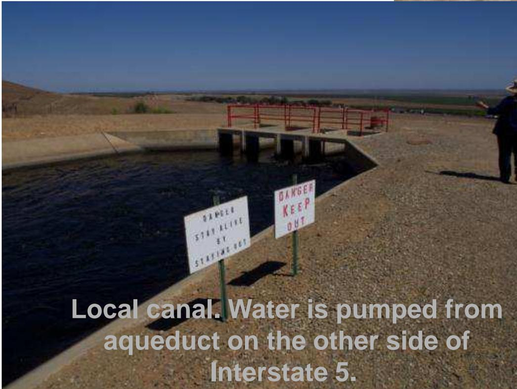
**Local canal. Water is pumped from aqueduct on the other side of Interstate 5.**
