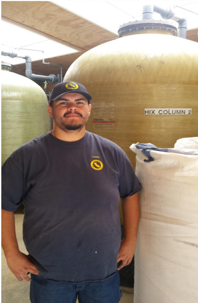
Cal Water treatment plant supervisor in Bodfish area of Kern Valley with vessels that filter contaminants from local groundwater including uranium, selenium, arsenic, and fluoride.
